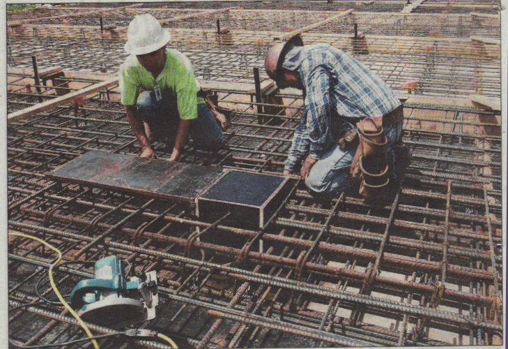
Christian Romero, left, and Jesus Medrano, both of West Palm Beach, use wire ties to reinforce the rebar for the exterior wall of the gymnasium under construction at Hillel Day School of Boca Raton. Staff photo/Kimberli DiMare
